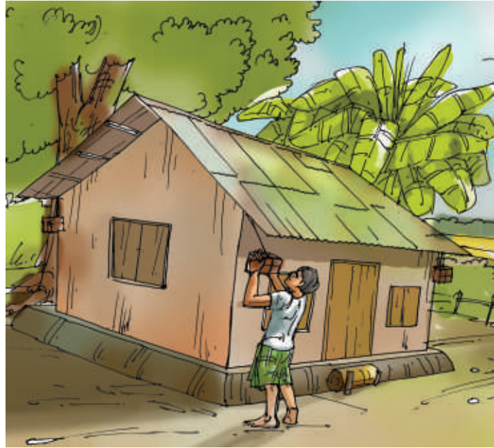
Hanging weights from the four corners of the roof during cyclone season
