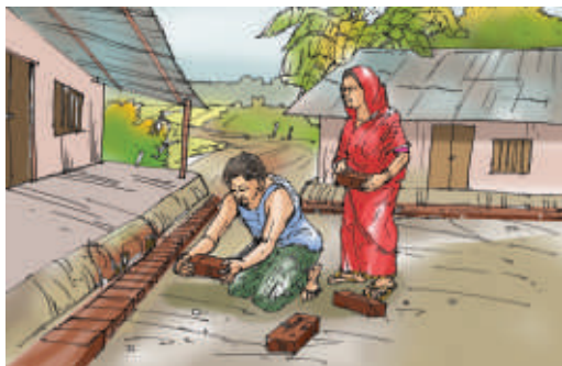
Laying bricks in a row to prevent damage to plinth area from rain water falling from roof
