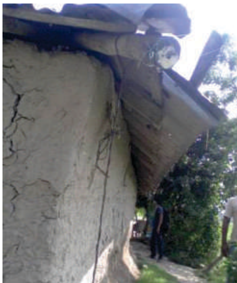
Mud walls with wooden pegs fixed on the ground
